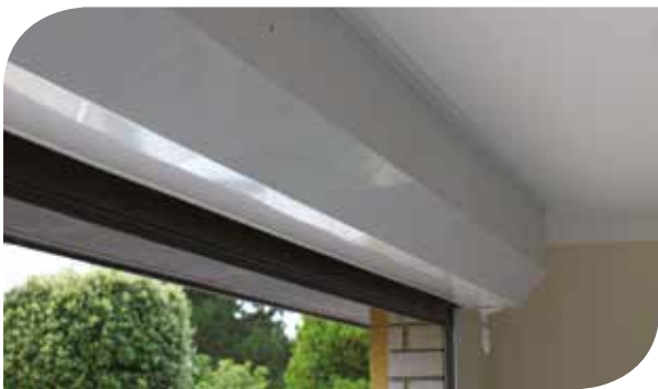
Internal view showing canopy (box)
